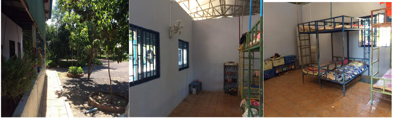
The completion of Boy building renovation, September 2016
